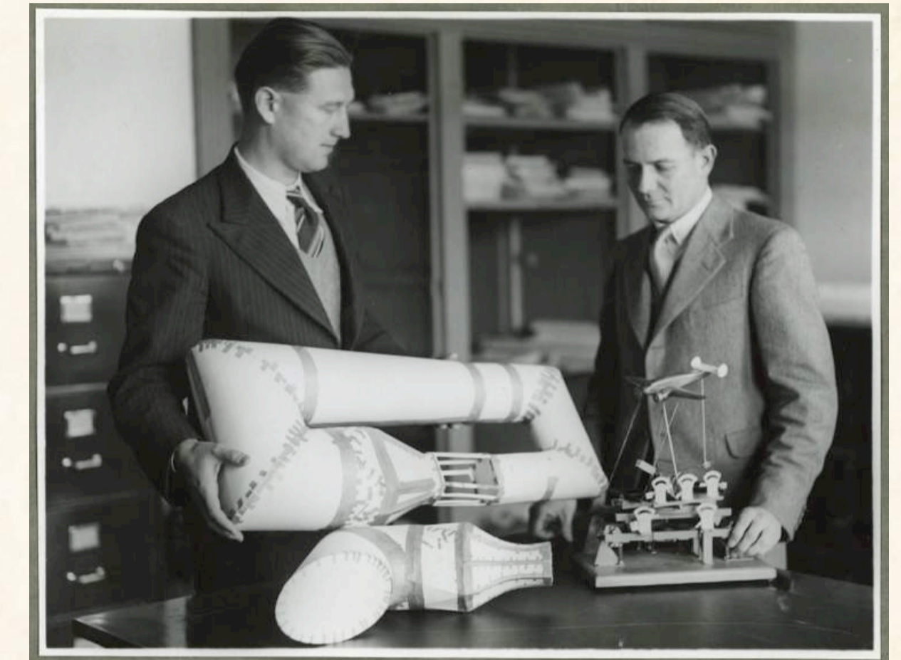
Construction of the wind tunnel commenced in 1945
