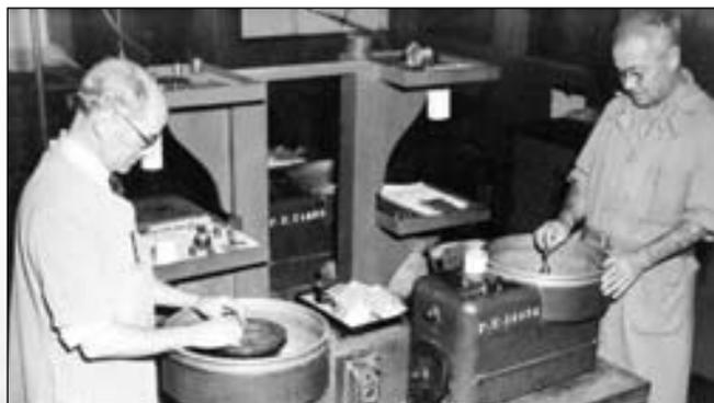
*Optical glass blanks being shaped for preparing lenses and prisms, c.1947.*
