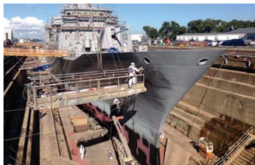
New Zealand ship being painted with Haze Grey paint originally developed by DSTO for the Royal Australian Navy.
