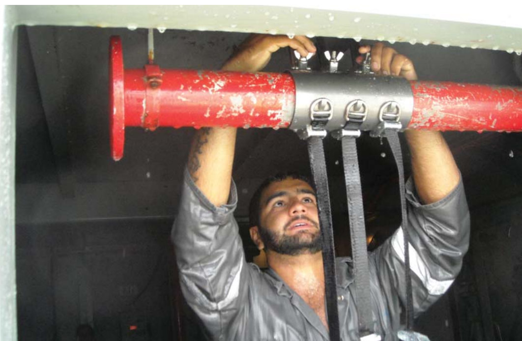
Innovative lever clamp being installed.
