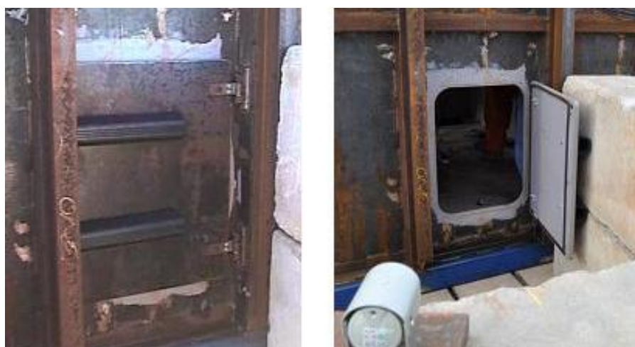
Figure 13: Trials structure vent hatch
