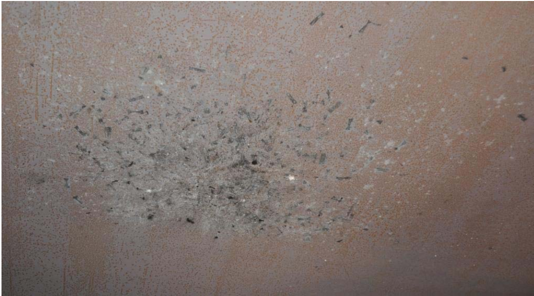
Figure 47: Propellant impact marks on the ceiling of the trials structure parallel to the chest and groin position of Person C, Experiment 1.
