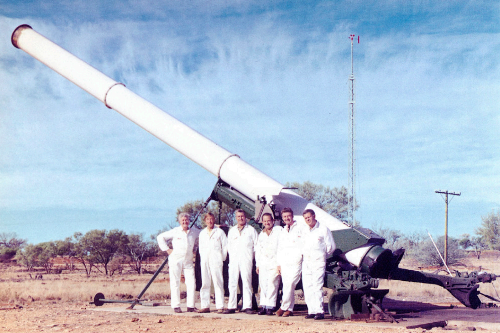
▲ The 10-metre-long launching tube of the Petrel supersonic rocket target, at its down-range site.
