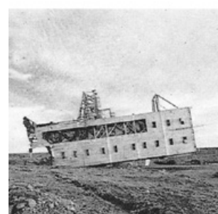
Toppling the Area 6 gantry tower prior to cutting it up for scrap.
