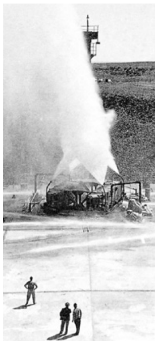
Above: Testing the firefighting system at the ELDO launcher. Such systems needed a large water storage capacity.
