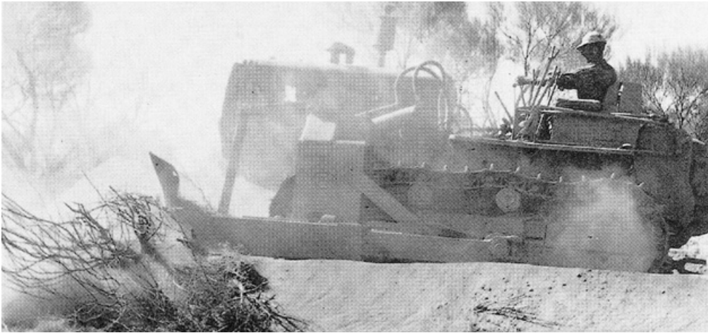
Grading one of Beadell's 'gunbarrel' roads.
