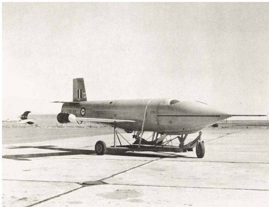
ARL undertook performance evaluations of the Mk 2 Jindivik, A92-60 on behalf of the RAAF, with a particular focus on the NACA submerged-type engine air intake. Woomera, circa 1958.
