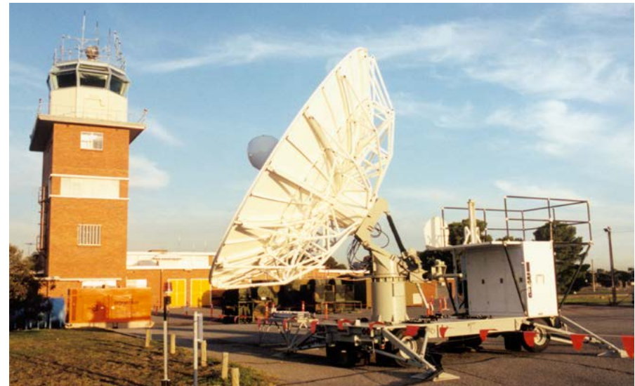
A Ku band satellite communications dish was installed at RAAF Edinburgh for in-flight adjustments to the carefully prepared Global Hawk flight plans as well as to receive radar and camera data from thousands of kilometres away.
