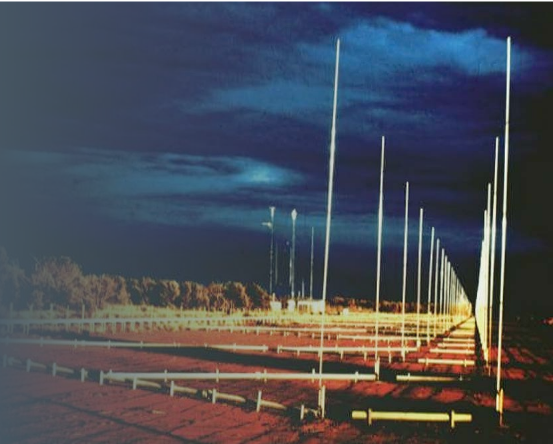
Jindalee Stage A receiver array near Alice Springs produced several narrow beams centred on the A76 international air route.
