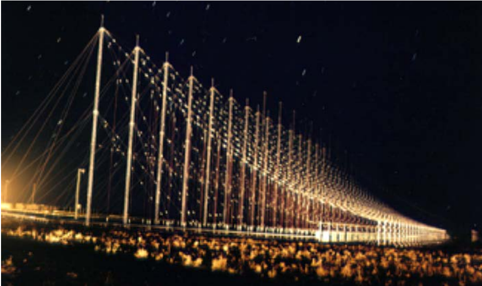
The Laverton transmit site used two orthogonal transmit antennas with a single set of transmitters that could be rapidly switched from one array to the other, while the Longreach radar used a single set of antennas.
