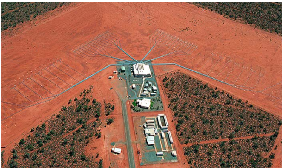
Laverton transmit array from the air.
