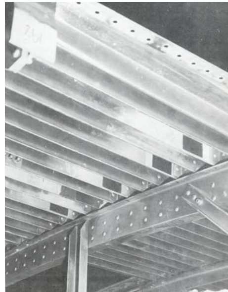
View of the boron/epoxy patches bonded over the cracks.
