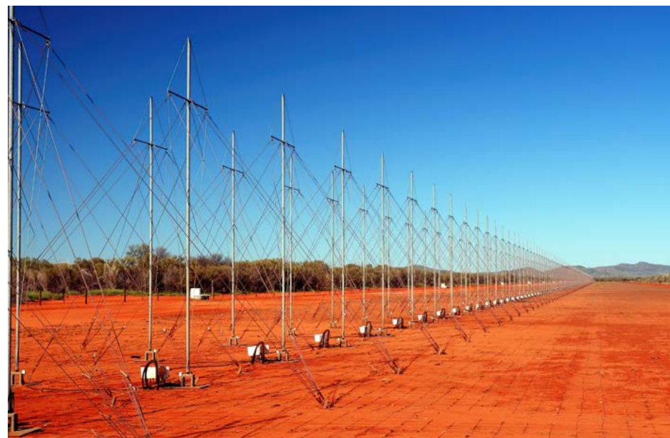
| The Jindalee Stage B receive array is 2.8 km long with 924 fan antennas and a copper mesh ground screen to enhance performance at low elevation angles.
